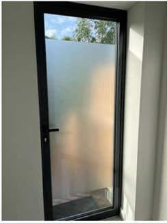
Dark grey, aluminium frame, double-glazed single door with black lever handle and cylinder lock
