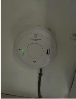
White plastic, carbon monoxide detector next to the boiler (top floor landing)
