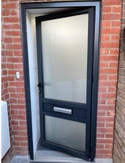
Dark grey aluminium frame, front door with 2x obscure double-glazed panes, black lever handle, 1x cylinder lock
